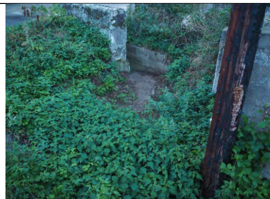
Figure 5 Traversée amont RD 1086
